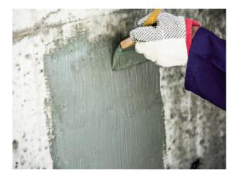
While the substrate is damp but free from standing water, apply the mixed product by medium hard short bristle brush, trowel or roller checking that the first coat is at a minimum wet film thickness of no more than 1.5mm and no less than 0.5mm. The product should always be finished in one direction.
